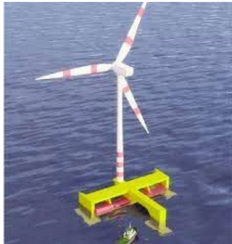
Floating power plant
